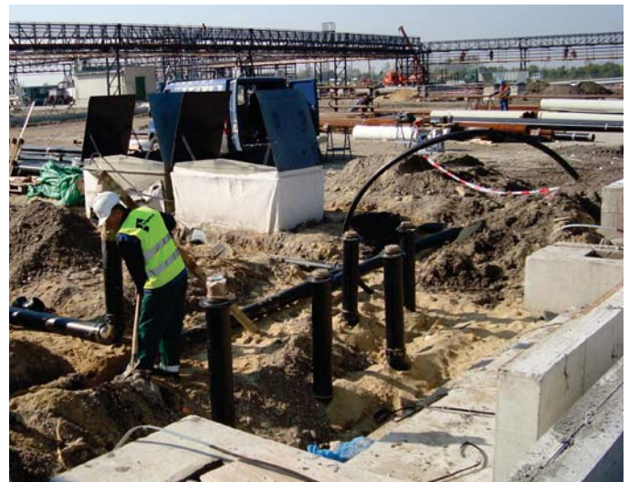
General view of construction site in October 2010
