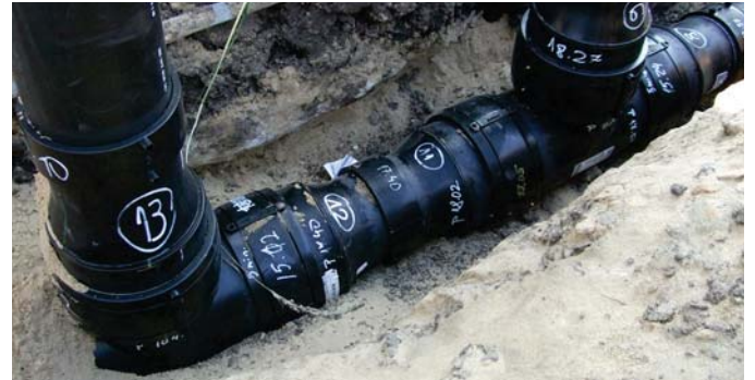
Close up of a 6" double wall elbow and tee
