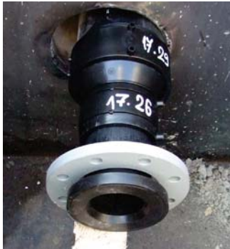
4" double wall flanged termination
