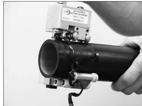
Scraping UPP Primary Pipe Using Scraping Tool
