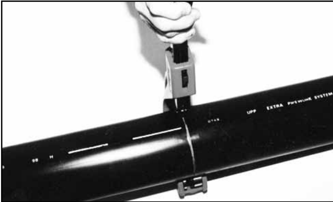
Cutting primary pipe using UPP cutting tool
