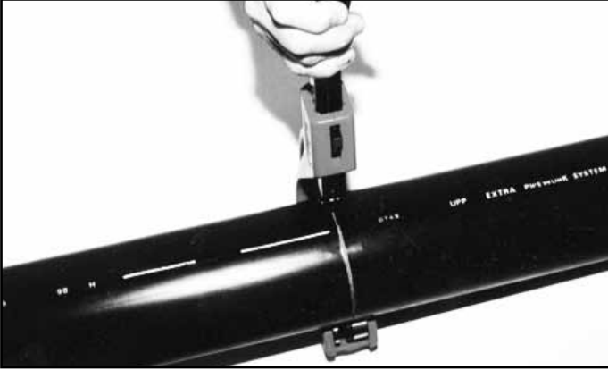
Cutting primary pipe using UPP cutting tool
