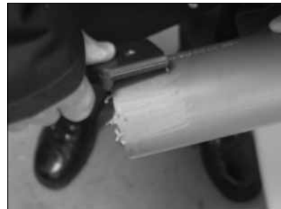
Scraping UPP Secondary Pipe Using Hand Scraper
