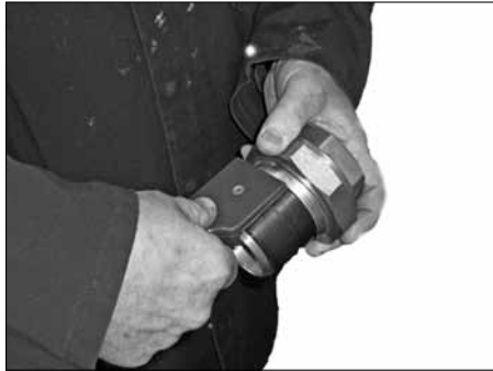
Scraping UPP Non-Electrofusion Fitting with Hand Scraper
