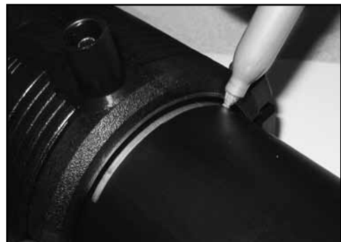
Marking Insertion Depth
