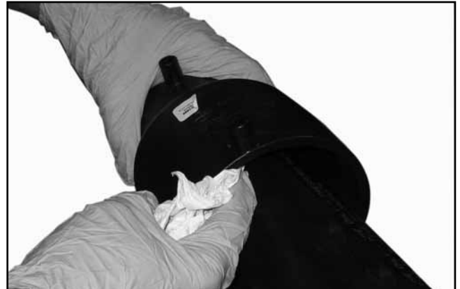
Clean Inside of Secondary
