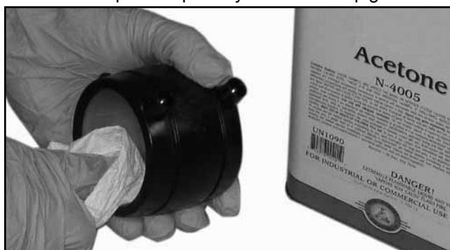
Clean Weld Coupler with Acetone
