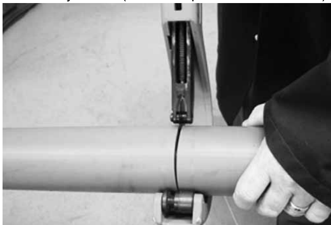
Cutting Secondary Pipe Using UPP Cutting Tool
