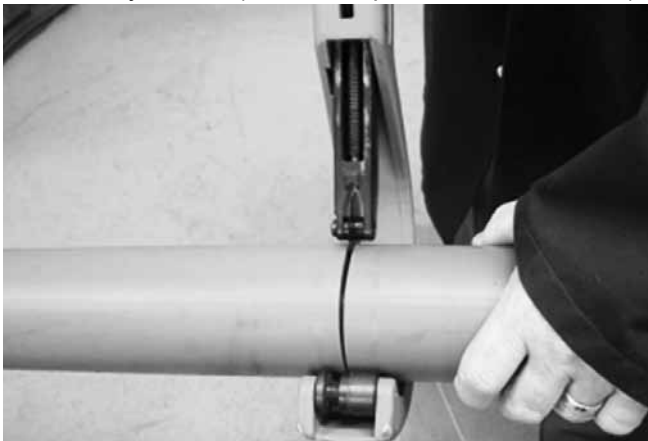
Cutting Secondary Pipe Using UPP Cutting Tool
