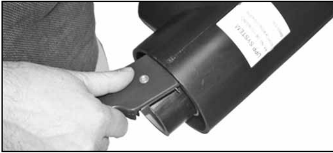
Scrape Primary and Secondary
