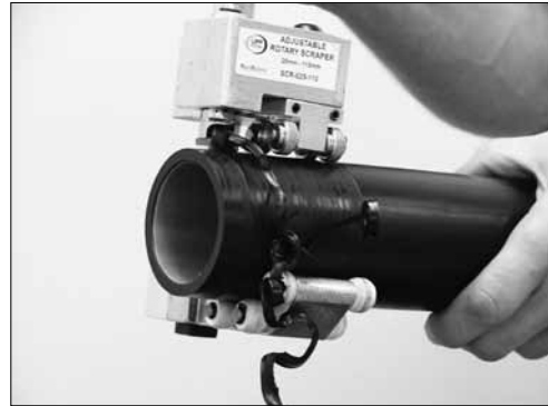
Scraping UPP Primary Pipe Using Scraping Tool
