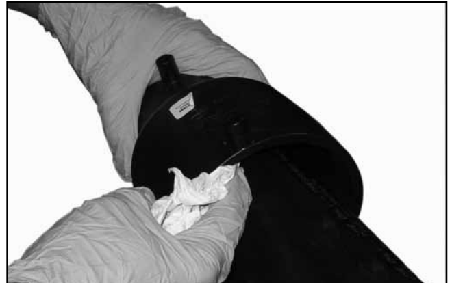
Clean Inside of Secondary
