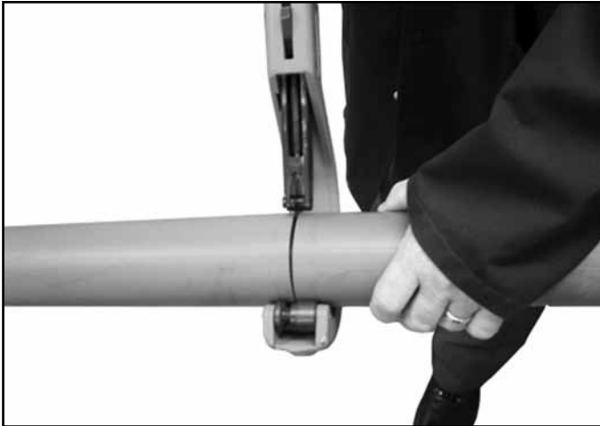
Cut Secondary Pipe
