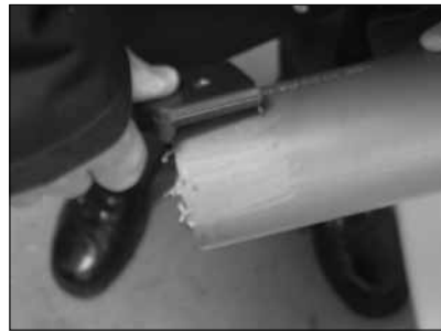
Scraping UPP Secondary Pipe Using Hand Scraper
