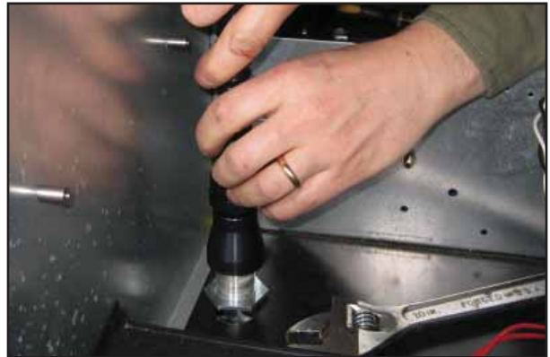
Figure 13: Attach Flexible Conduit
