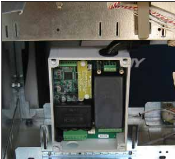
Figure 11: 90-degree Fitting Installed
