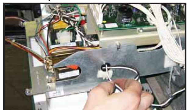
Figure 10: Power Harness Wiring
