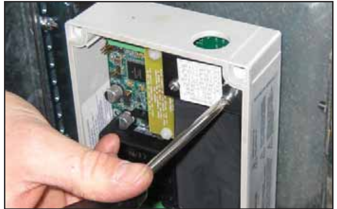
Figure 12: Remove Wiring Cover
