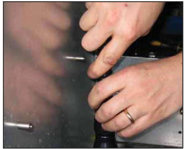
Figure 11: Flexible Conduit Installation
