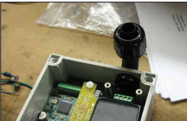
Figure 7: 90-Degree Fitting Installed
