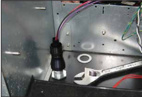
Figure 6: Straight Conduit Installed
