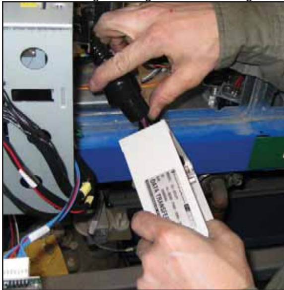
Figure 12: Pull wires through 90-degree fitting
