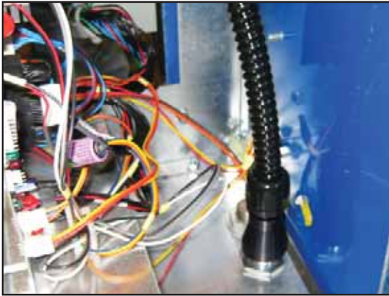
Figure 11: Flexible Conduit Connected
