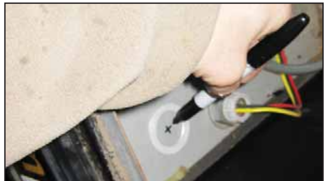
Figure 5: Mark Drilling Location
