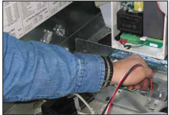
Figure 8: Pulling Wires Through Opening
