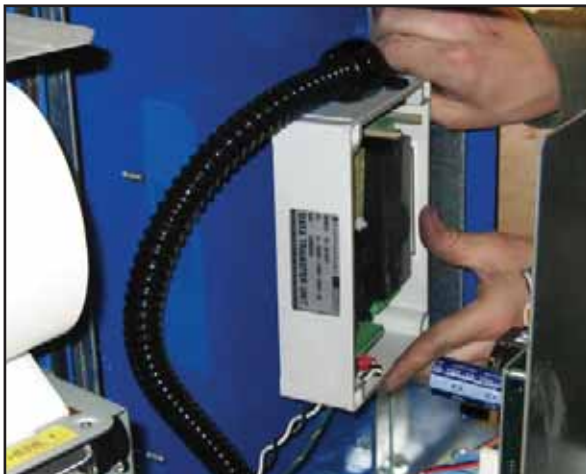
Figure 13: 90-Degree Conduit Connected
