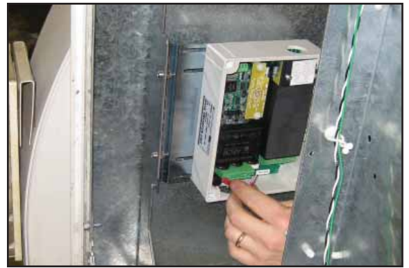
Figure 3: Attach DTU to Dispenser
