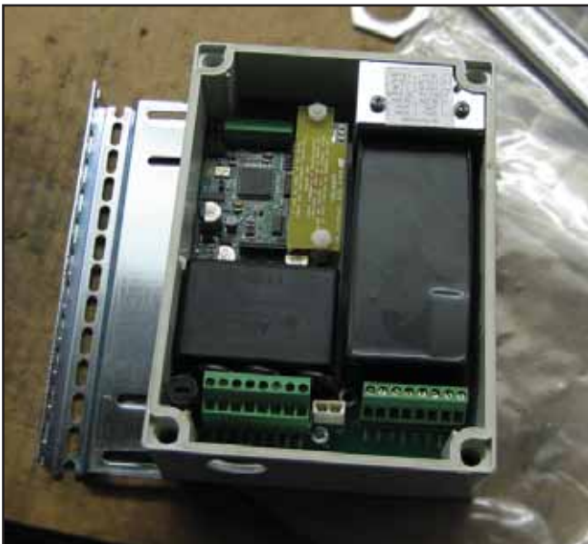
Figure 2: Mounting Bracket Installed
