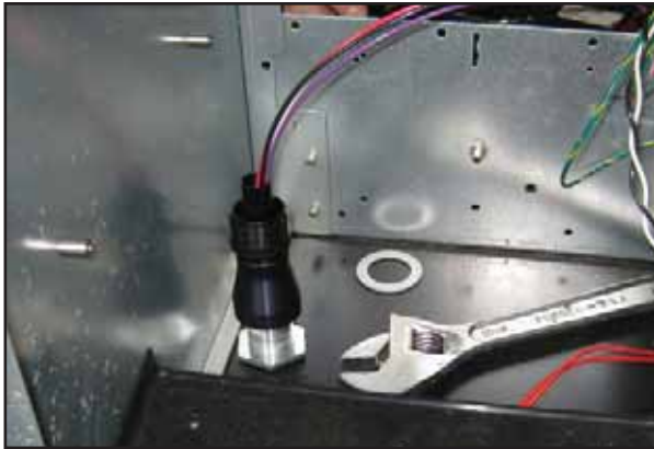
Figure 5: Straight Conduit Installed
