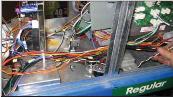
Figure 16: Power Cable Installation
