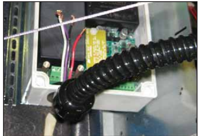
Figure 12: 90-Degree Fitting Installed
