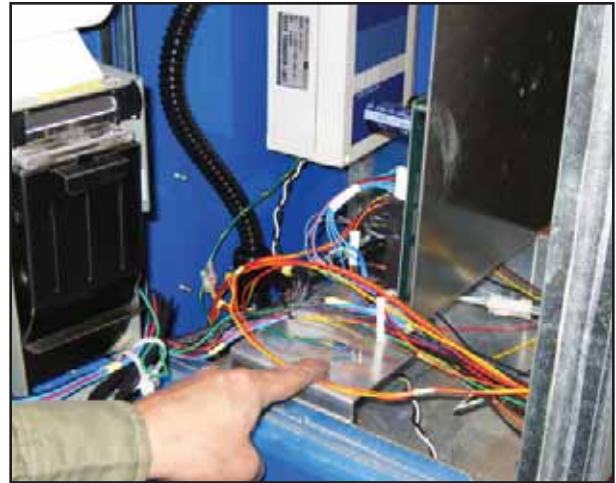
Figure 18: Ground Wire Attached
