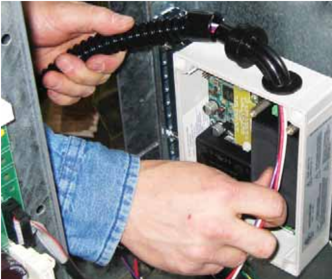
Figure 15: Attach Flexible Conduit to 90-Degree Fitting
