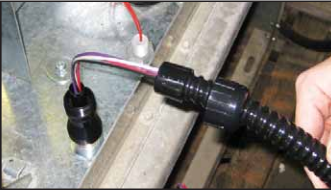
Figure 14: Attach Flexible Conduit to Potted Nipple
