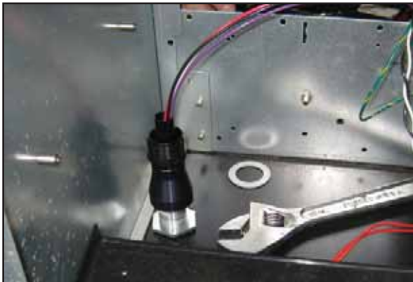
Figure 6: Straight Conduit Installed
