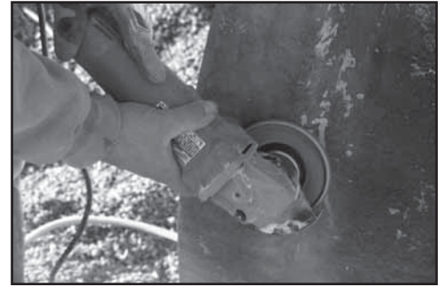
Figure 2 - Sanding the Sump
