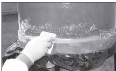
Figure 5 - Smoothing Catalyzed Putty
