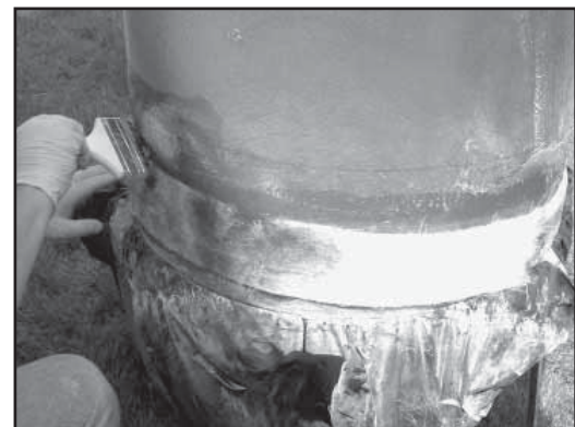
Figure 9 - Saturating with Resin
