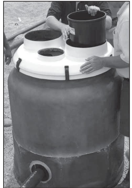
Figure 3 Aligning Multi-Port Sump Shield
