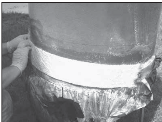
Figure 8 - Applying Mat
