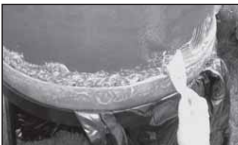
Figure 4 - Applying Catalyzed Putty
