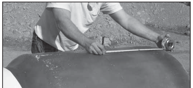
Figure 1 - Marking the Sump for Cutting
