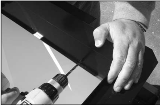
Figure 7 - Drilling from the Inside of the Sump
