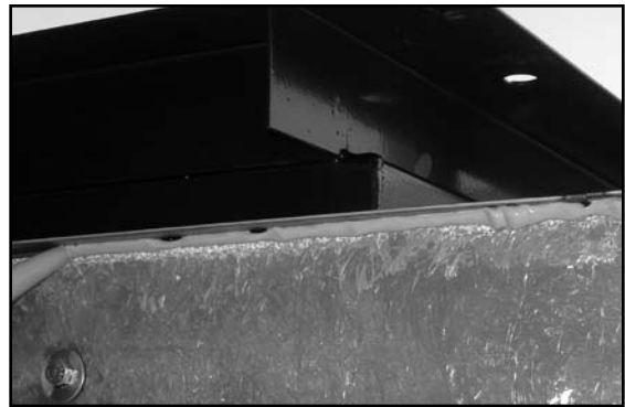
Figure 27 - Applying Sealant to Sump Top
