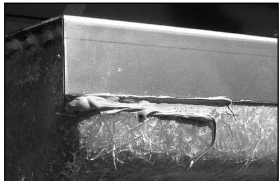
Figure 11 - Sealed Sump Top
