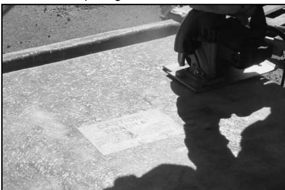
Figure 14 - Cutting Down Sump
