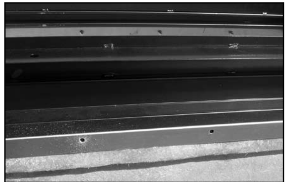
Figure 5 - Matching Up Guide Holes
