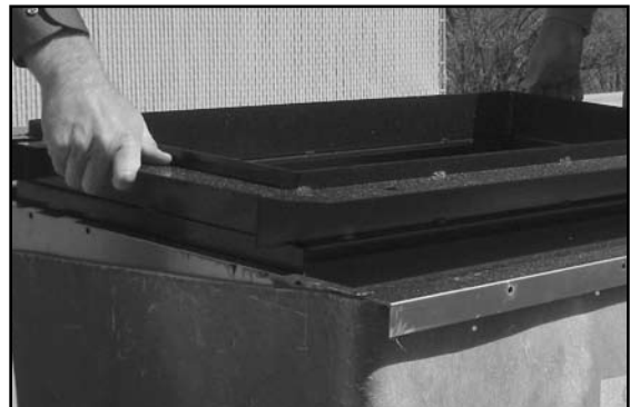
Figure 16 - Installing Metal Top
