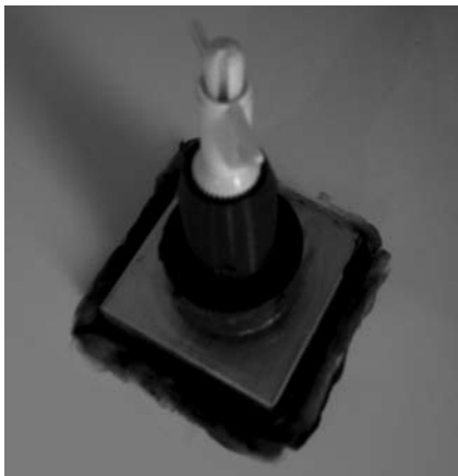
Figure 37 - Plug in Monitoring Fluid Port
