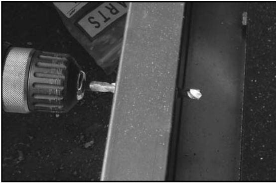
Figure 18 - Drilling Through Metal Frame
