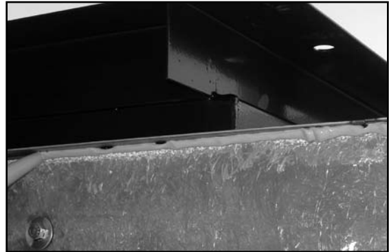
Figure 10 - Applying Sealant to Sump Top
