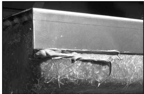
Figure 28 - Applying Sealant to Sump Top
