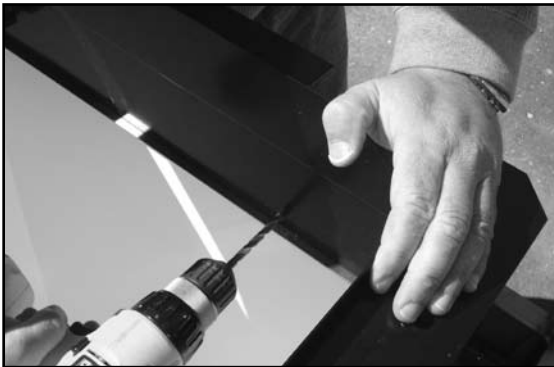
Figure 24 - Drilling from the Inside of the Sump
