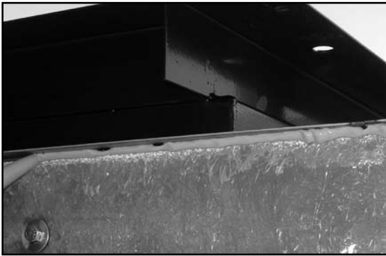
Figure 34 - Applying Sealant to Sump Top
