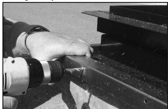
Figure 17 - Drilling Through Guide Holes
