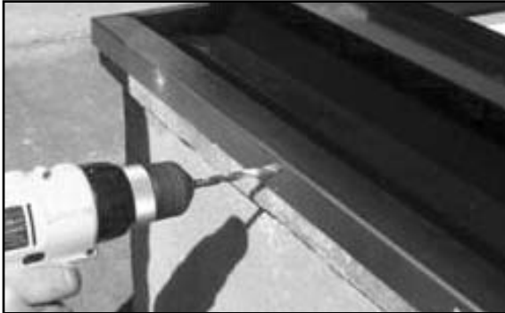
Figure 1 - Drilling into Metal Frame
