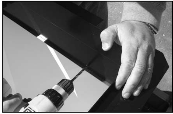
Figure 31 - Drilling from the Inside of the Sump
