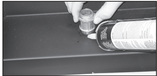
Figure 4: Seal Grommet Area
