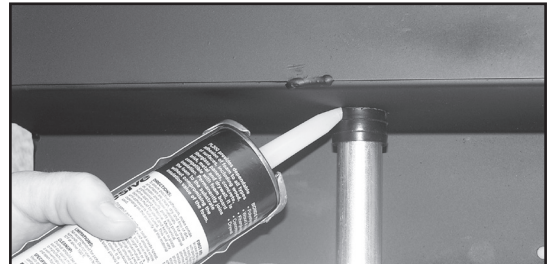
Figure 5: Seal Under Grommet
