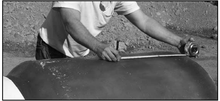
Figure 12 - Marking the Sump for Cutting
