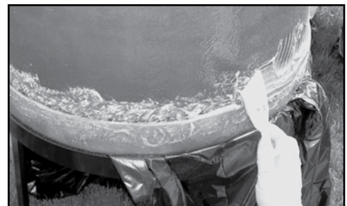
Figure 4 - Applying Catalyzed Putty
