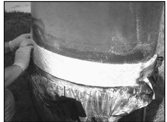
Figure 8 - Applying Mat
