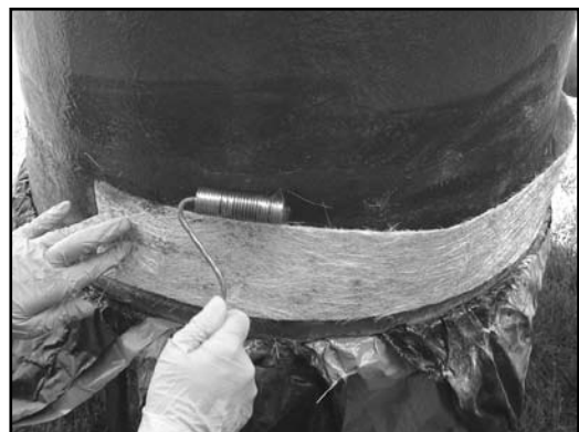
Figure 11 - Applying 2 nd Layer
