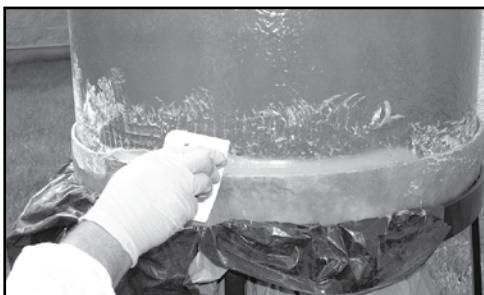
Figure 5 - Smoothing Catalyzed Putty
