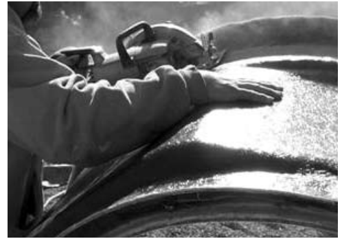
Figure 1 - Removing Bottom Ring
