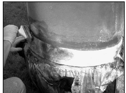
Figure 9 - Saturating with Resin
