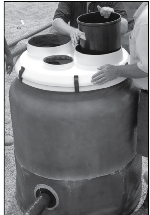
Figure 3 Aligning Multi-Port Sump Shield
